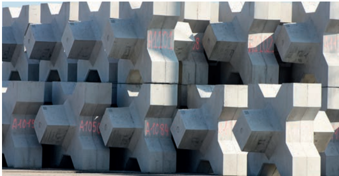
The Xbloc® is a concrete block with high reliability used for the construction of the breakwater. It will be the emblem of the worksite. The Xbloc® has a high level of design and those used on site will reach nearly 4 meters in height.
